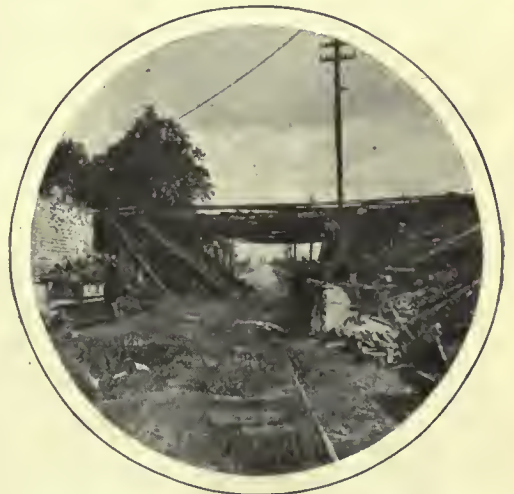
THE BROKEN RAILWAY BRIDGE AT TERGNIER.
