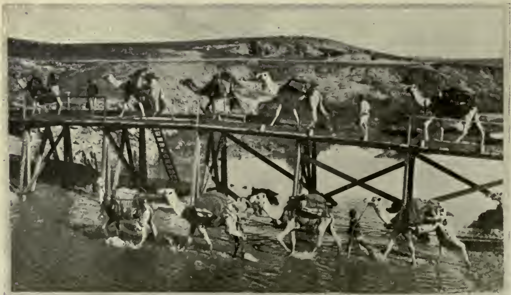
A TRESSEL BRIDGE BUILT BY ANZAC ENGINEERS.
