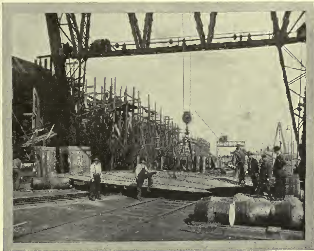
LIFTING INTO POSITION A LARGE FABRICATED SECTION OF A STEAMER.
