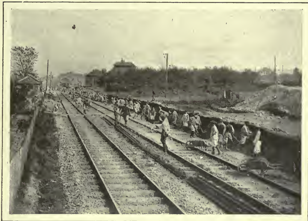
CHINESE LABOURERS DOUBLING A RAILWAY LINE. [French official photograph.]
