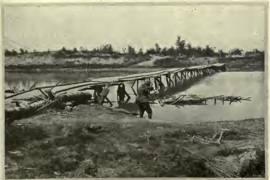
AUSTRIAN BRIDGE ON THE OLD PIAVE.
