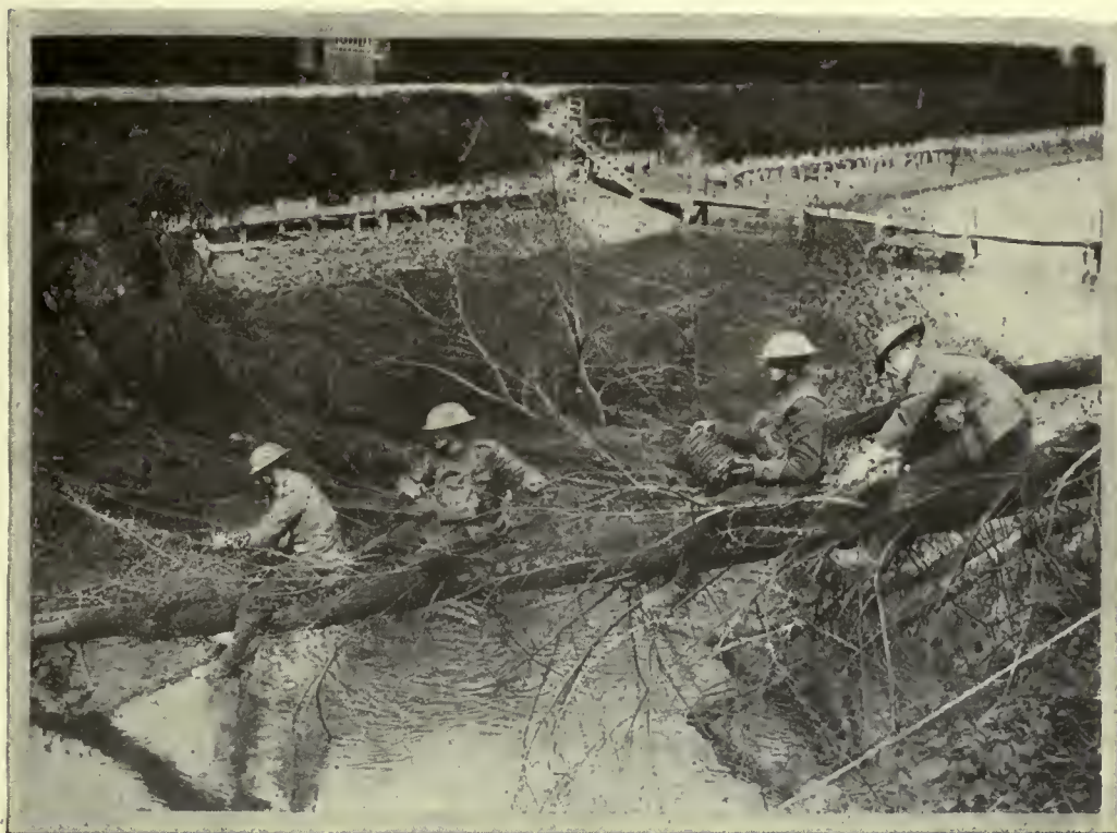
WIRING TREES FELLED ACROSS A CANAL TO HOLD UP THE ENEMY.
