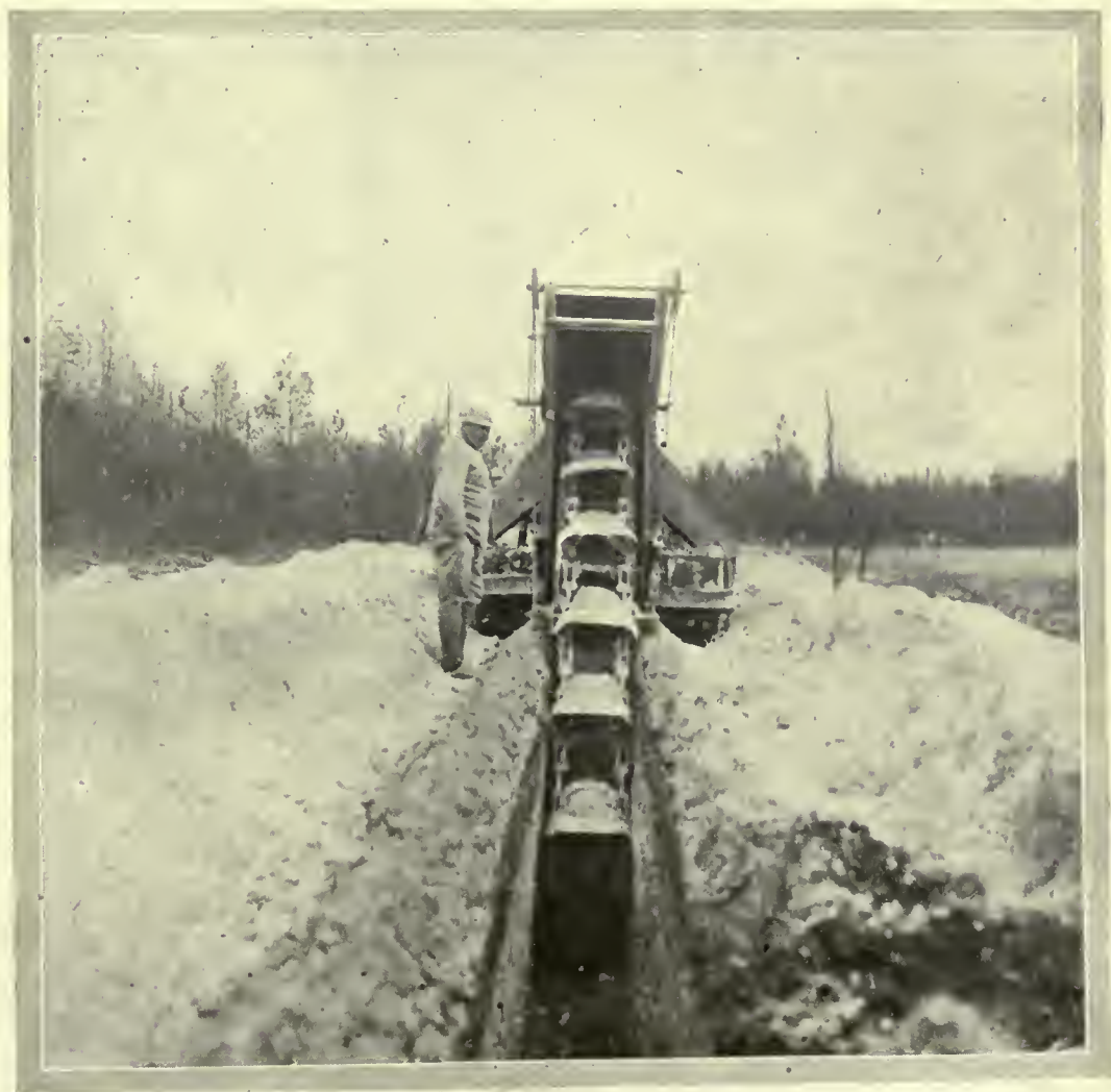
FRENCH TRENCH-DIGGING MACHINE.
