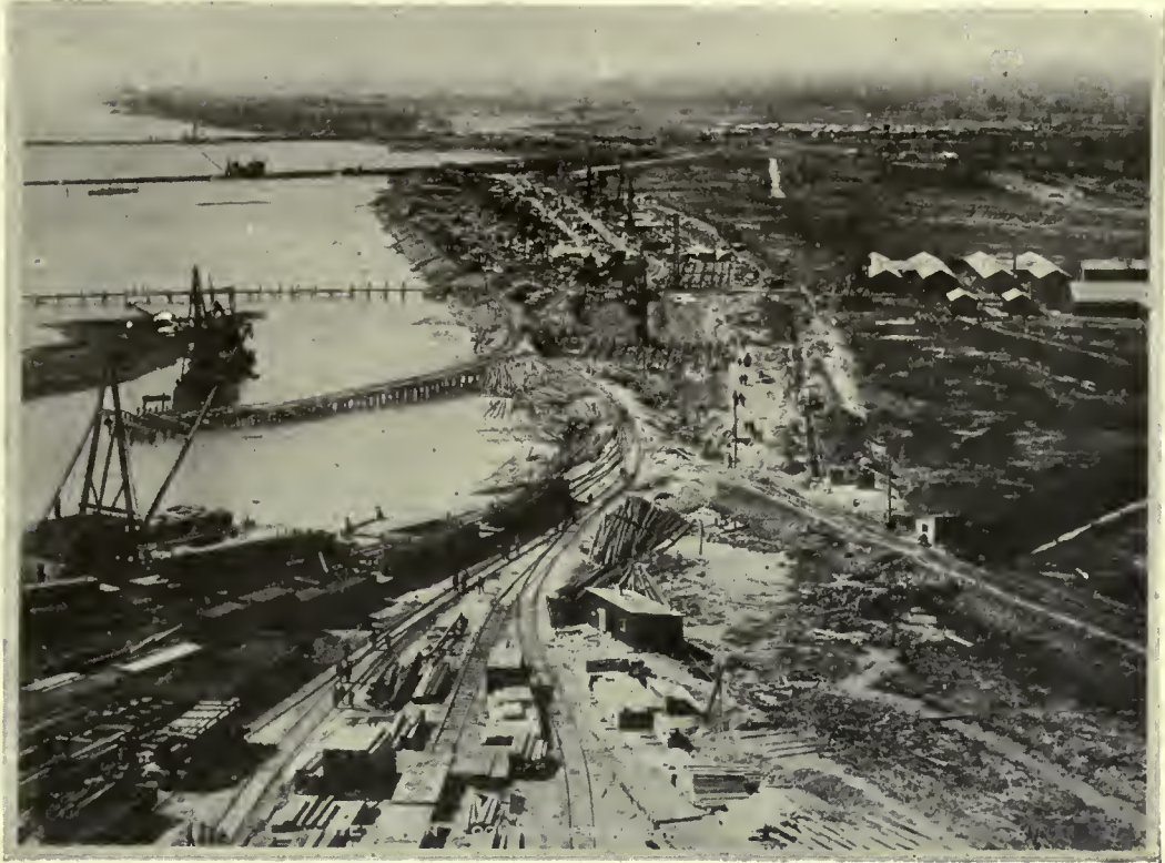
HOG ISLAND AFTER THIRTY WEEKS' WORK: THE WET DOCK BASINS.
